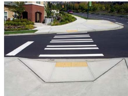
The corner pictured above (top) has an incomplete sidewalk and no curb ramp, forcing some pedestrians to go around, either onto a busy street, or into a parking lot in order to cross the intersection. The other corner pictured above (bottom) with curb ramps and crosswalk is much more safe and accessible.
