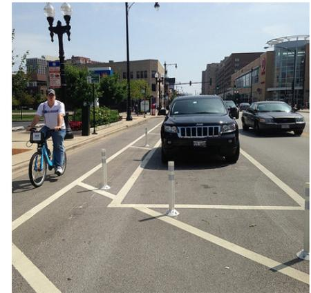
*Above:* Move the paint to create 10 foot travel lanes, which allows the additional pavement to be reallocated for other uses, such as parking and bike lanes, as seen in downtown Charlotte, NC (left) and Chicago, IL (right).
